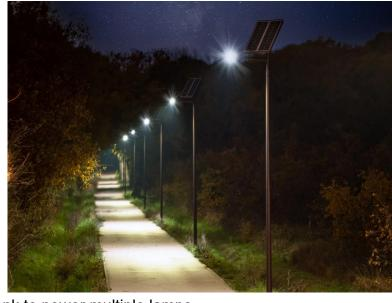
large central solar panel and battery bank to power multiple lamps.
